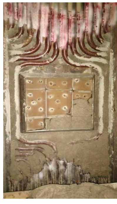
Door after application of Plastic Refractory from Inside Furnace
