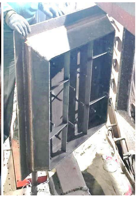
Door Before Application of Plastic refractory
