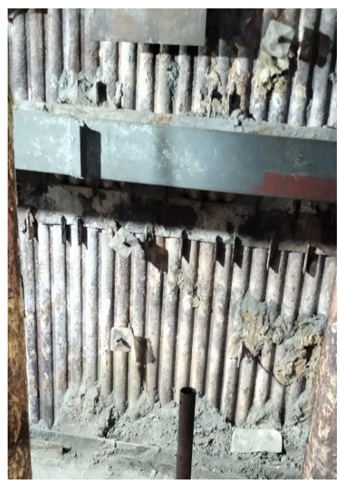
Before Cutting of Waterwall Tubes for manhole Bends Fit up & Welding
